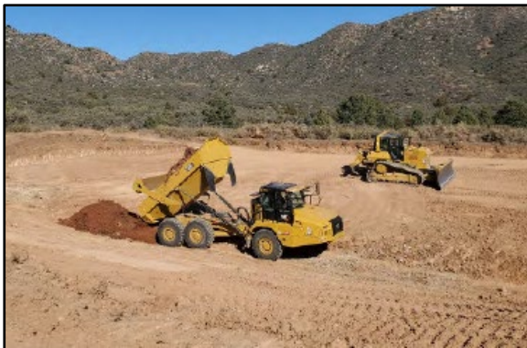
Placing mine waste into Junction Consolidation cell
